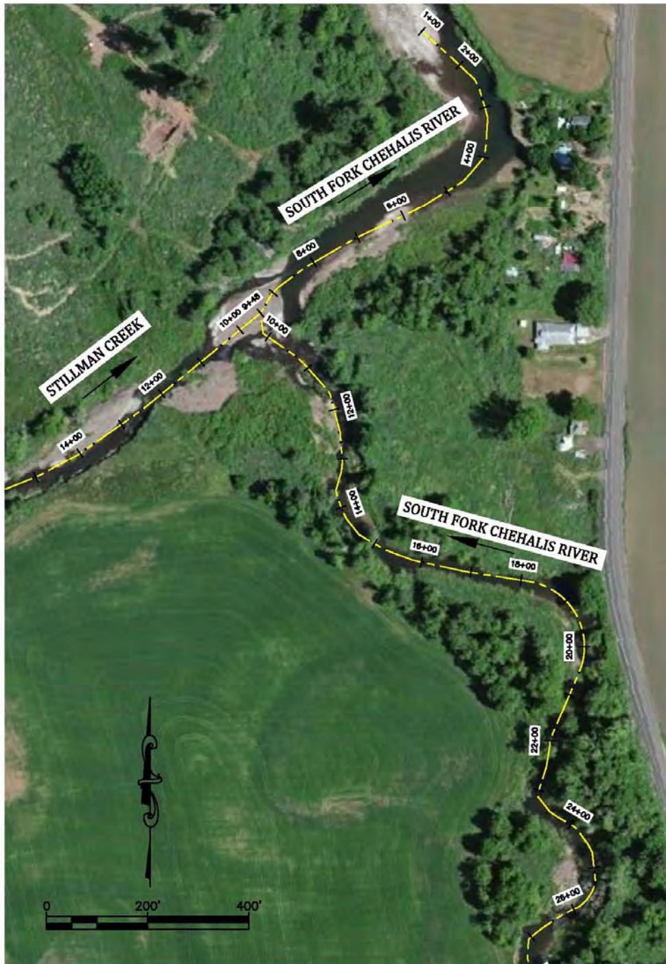
Figure 2. Aerial view of project reach and stream channel centerline.
