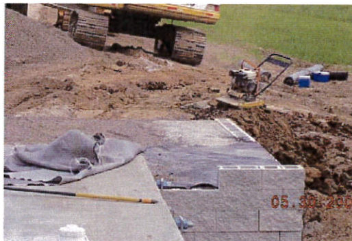
Figure 75. Photo. Parapet and wing wall construction, view 2.
