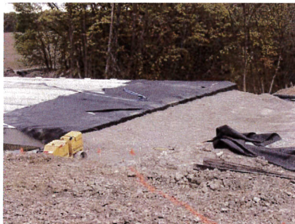
Figure 80. Photo. Second 6-inch fill lift.
