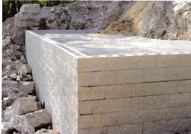
Figure 57. Photo. Right-angle wall corner.
