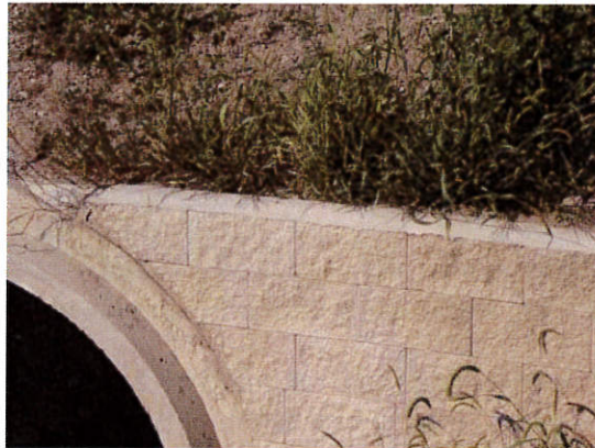
Figure 62. Photo. Square coping cap.
