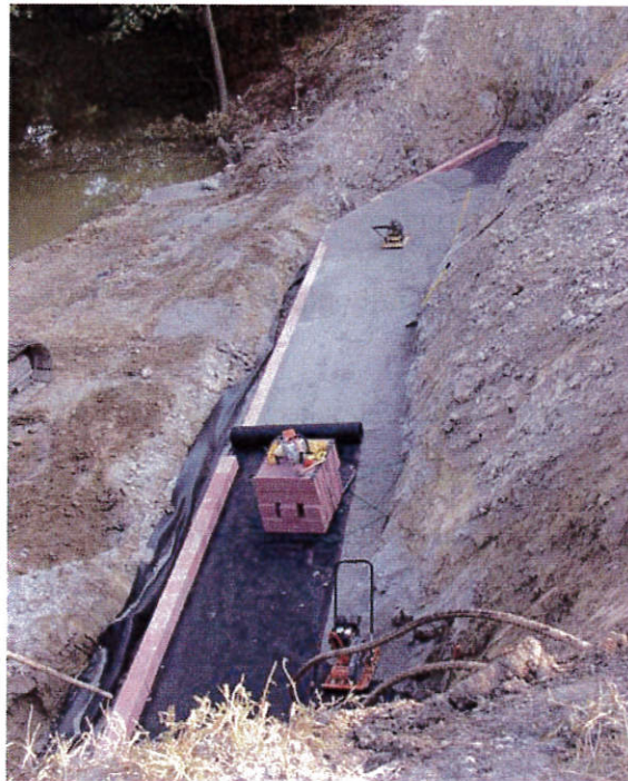
Figure 51. Reinforcement rolled out parallel to wall face.
