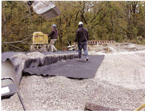
Figure 78. Photo. Secondary reinforcement sheet.
