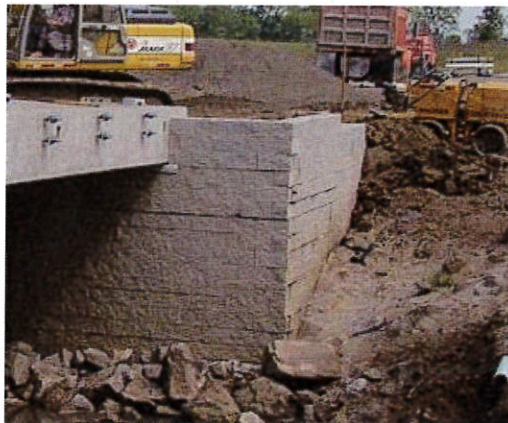
Figure 74. Photo. Parapet and wing wall construction, view 1.
