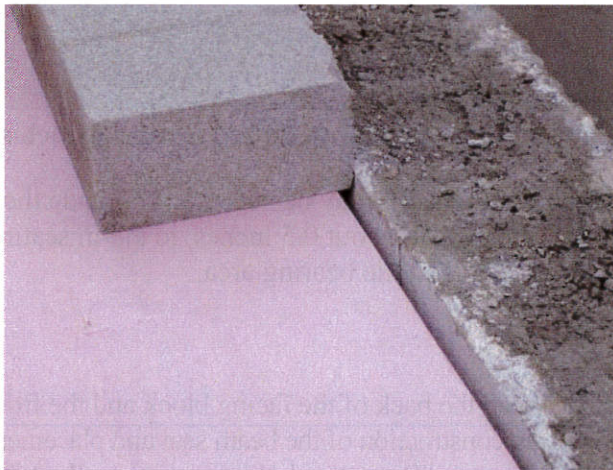
Figure 67. Photo. 4-inch concrete block on top of foam board against top CMU face block.
