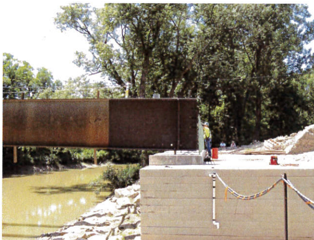
Figure 71. Photo. Steel girder on CIP footing.
