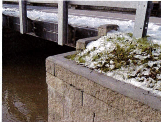
Figure 61. Photo. Rounded coping cap.
