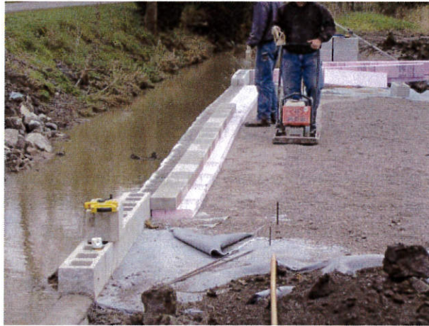
Figure 66. Photo. Foam board and 4-inch block assembly to form beam seat.
