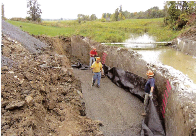
Figure 45. Photo. Building the RSF behind an existing abutment.
