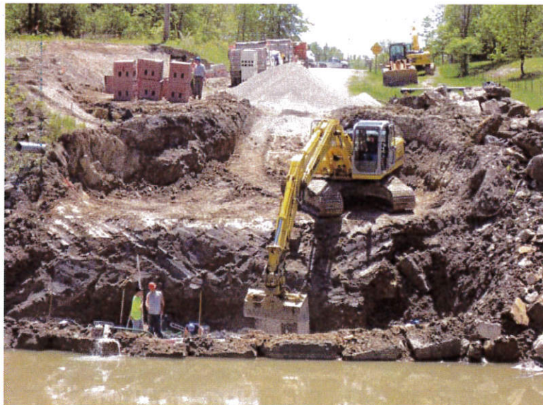
Figure 46. Photo. RSF excavation below stream level.
