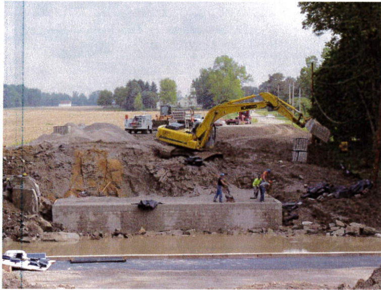
Figure 42. Photo. Horseshoe-shaped excavation with native soil still intact in middle.
