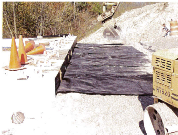
Figure 79. Photo. Completed wrapped approach layer.
