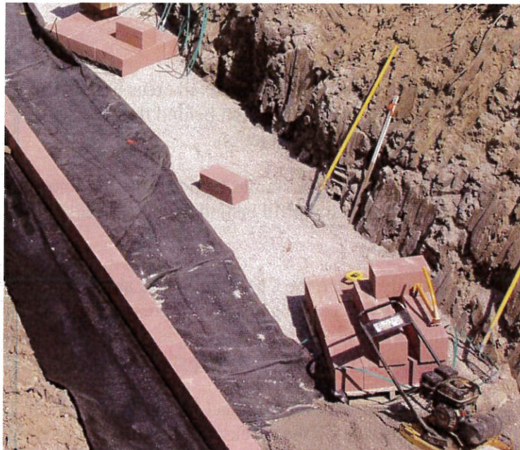
Figure 49. Photo. Placement of wall block on wrapped RSF.
