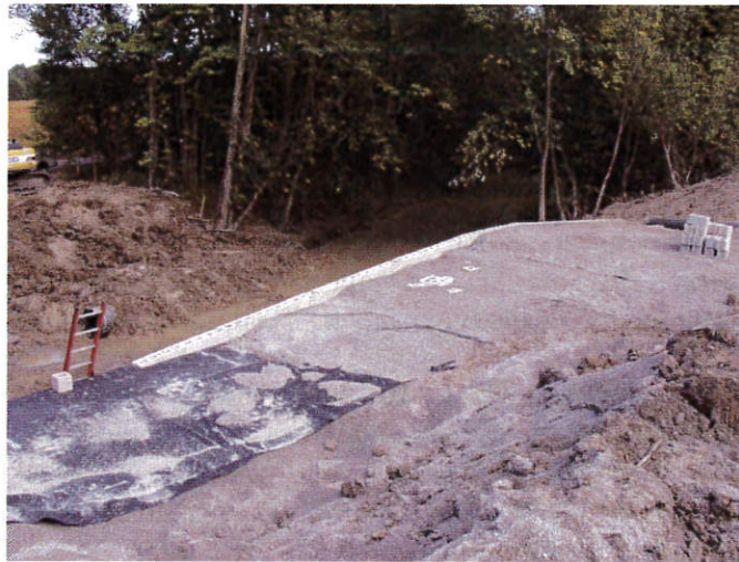
Figure 53. Photo. Superelevation reinforcement layers.
