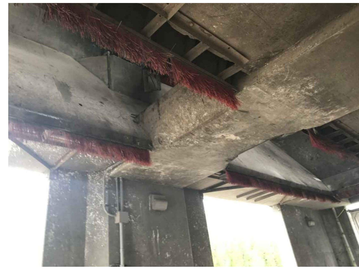
TYP CRANE BEAM DAMAGE DETAIL 1 - N.T.S.
