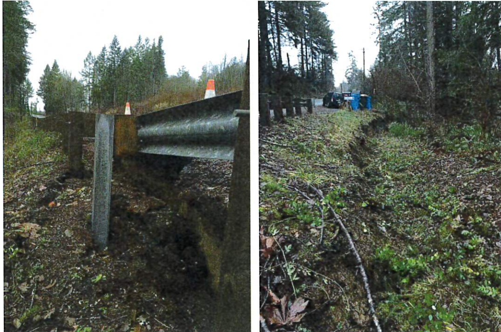
Photo 2. [Left] Looking west at scarp from below/south. [Right] Looking east along scarp
