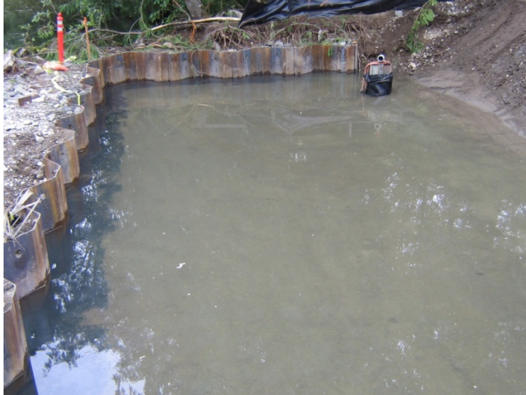
Figure 49. Photo. Sheet-pile supported excavation.
