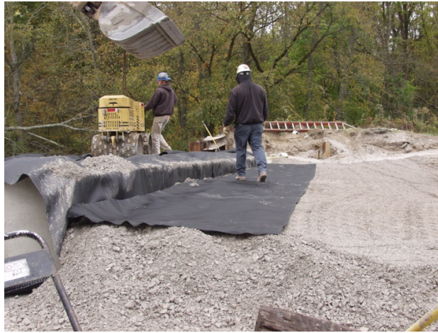
Figure 94. Photo. Secondary reinforcement sheet.
