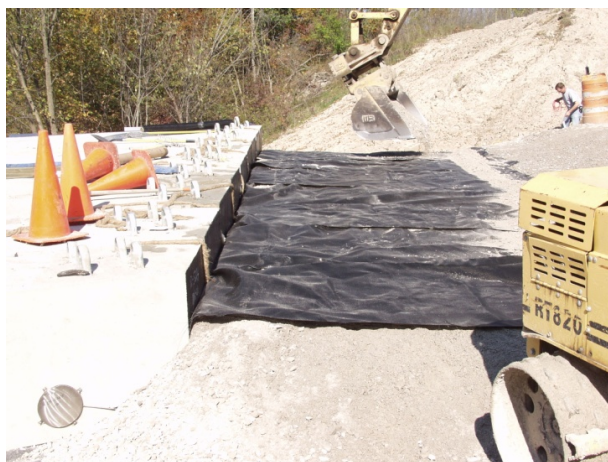
Figure 94. Photo. Secondary reinforcement sheet.
