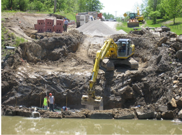
Figure 53. Photo. RSF excavation below the stream level.
