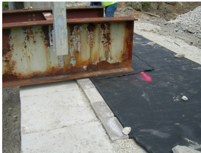
Figure 84. Photo. Additional reinforcement under the beam.
