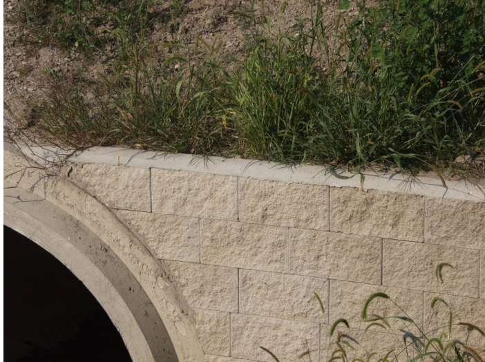
Figure 76. Photo. Rounded coping cap.
