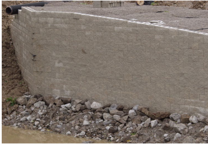
Figure 65. Photo. Blocks trimmed to match superelevation.
