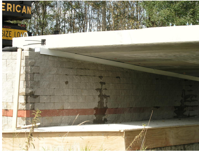
Figure 85. Photo. Aluminum flashing (drip edge) between the beams and the top of the CMU facing.
