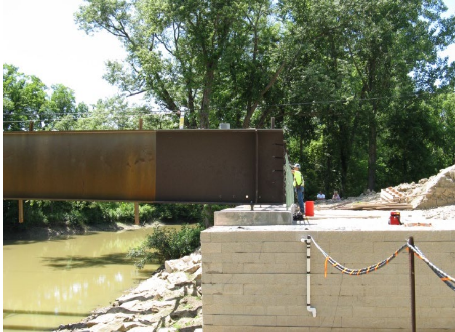
Figure 86. Photo. Steel girder on CIP footing.
