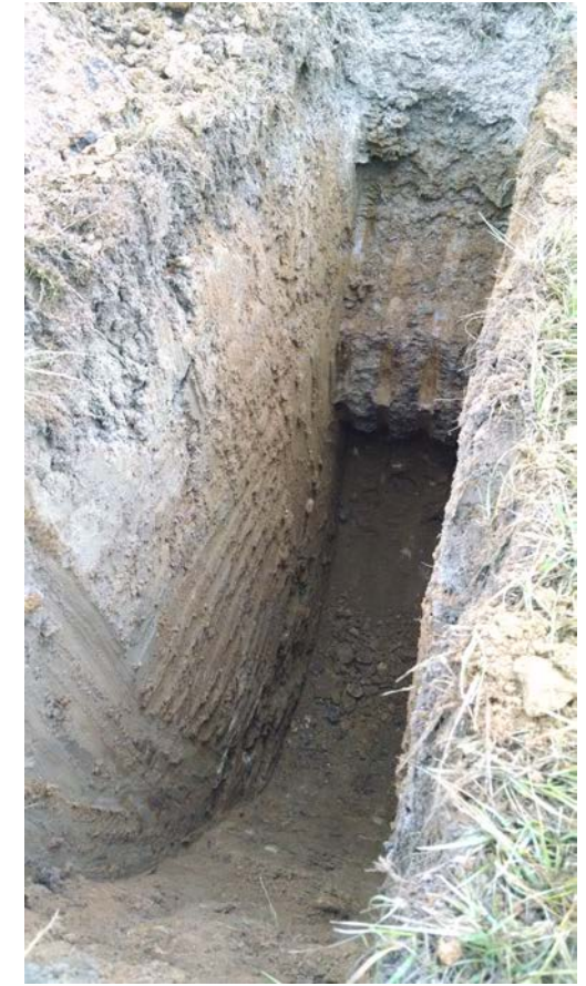
PHOTO OF EAST SIDE OF PIT
