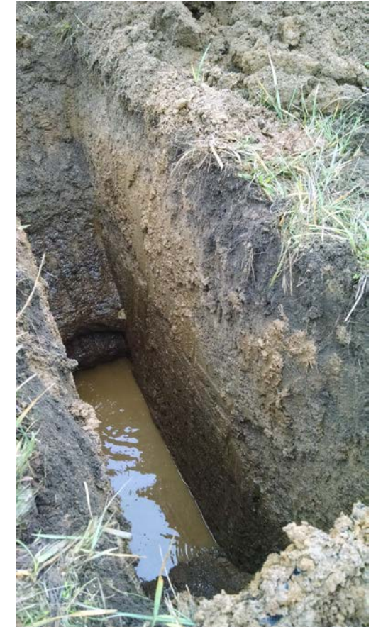
PHOTO OF WEST SIDE OF PIT
