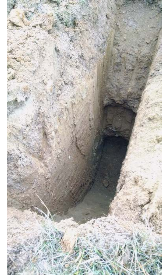
PHOTO OF EAST SIDE OF PIT
