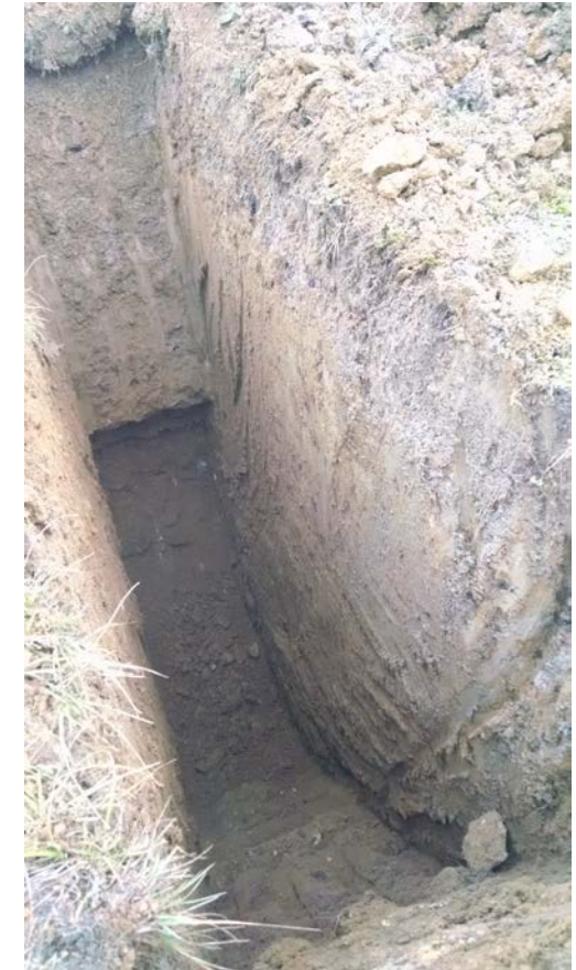
PHOTO OF WEST SIDE OF PIT
