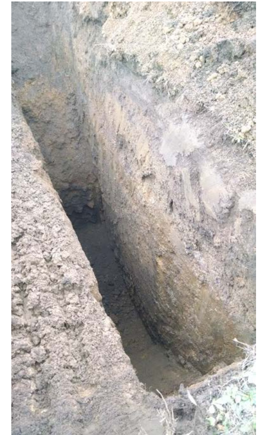
PHOTO OF WEST SIDE OF PIT
