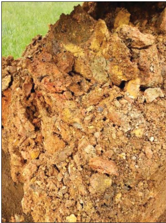
Photos TP-2: Test Pit TP-2 at approximately 8 feet in depth (below); Sample from bottom of exploration at 8 feet (left)
