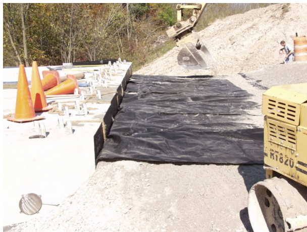
Figure 94. Photo. Secondary reinforcement sheet.
