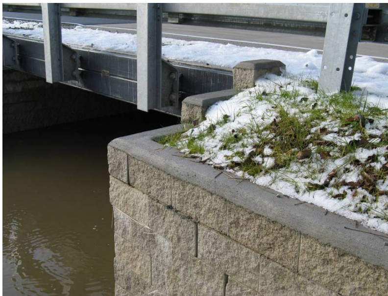
Figure 75. Photo. Square coping cap.
