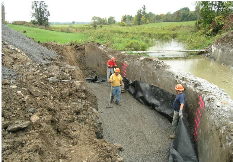
Figure 52. Photo. Building the RSF behind an existing abutment.
