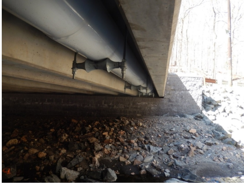
Figure 100. Photo. Utilities through a GRS abutment.
