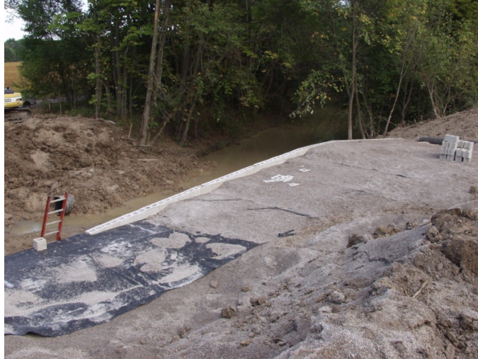
Figure 62. Photo. Superelevation reinforcement layers.
