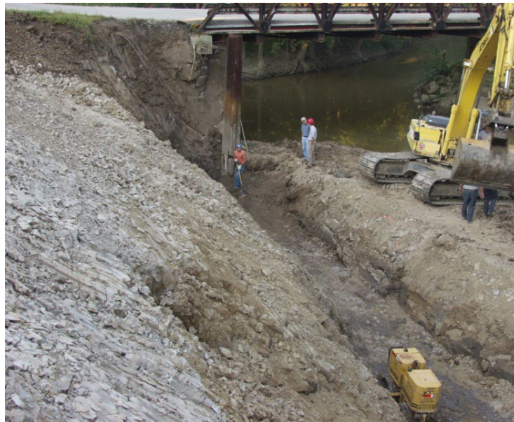
Figure 54. Photo. RSF cut preparation.
