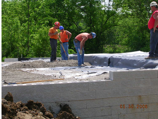
Figure 93. Photo. First 6-inch-thick fill lift.
