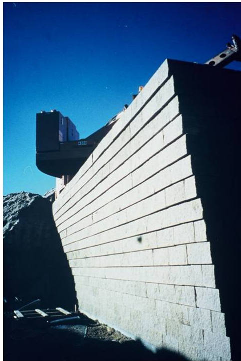
Figure 64. Photo. Negative batter wall face.
