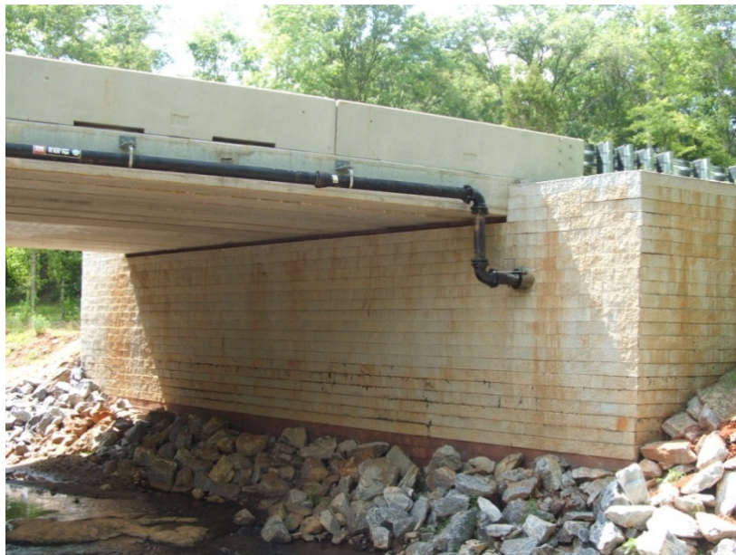
Figure 100. Photo. Utilities through a GRS abutment.
