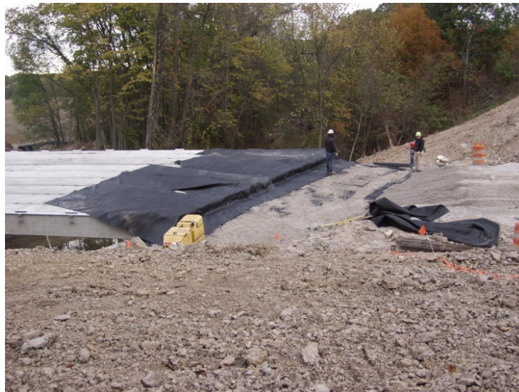
Figure 92. Photo. Reinforcement placement.
