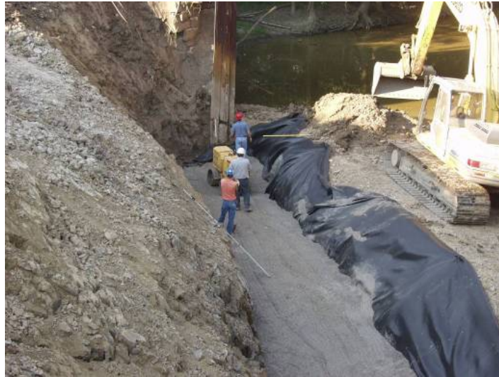
Figure 55. Photo. Encapsulation of fill in RSF.
