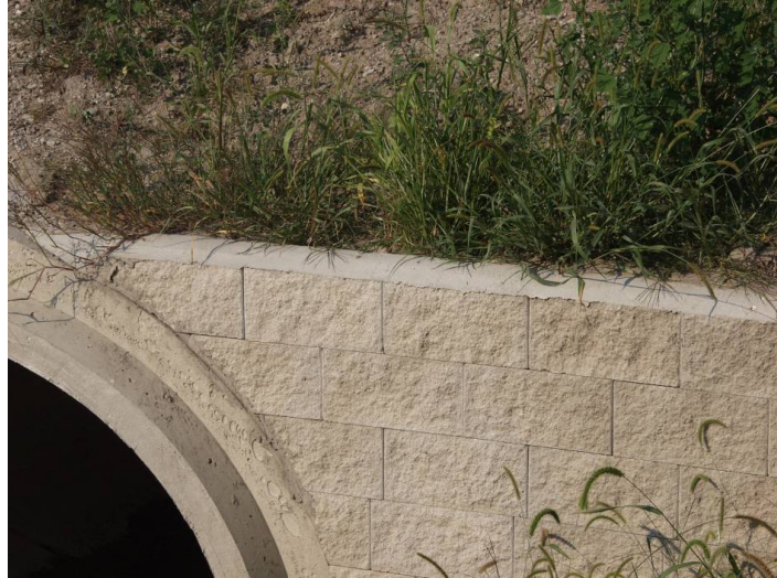
Figure 76. Photo. Rounded coping cap.
