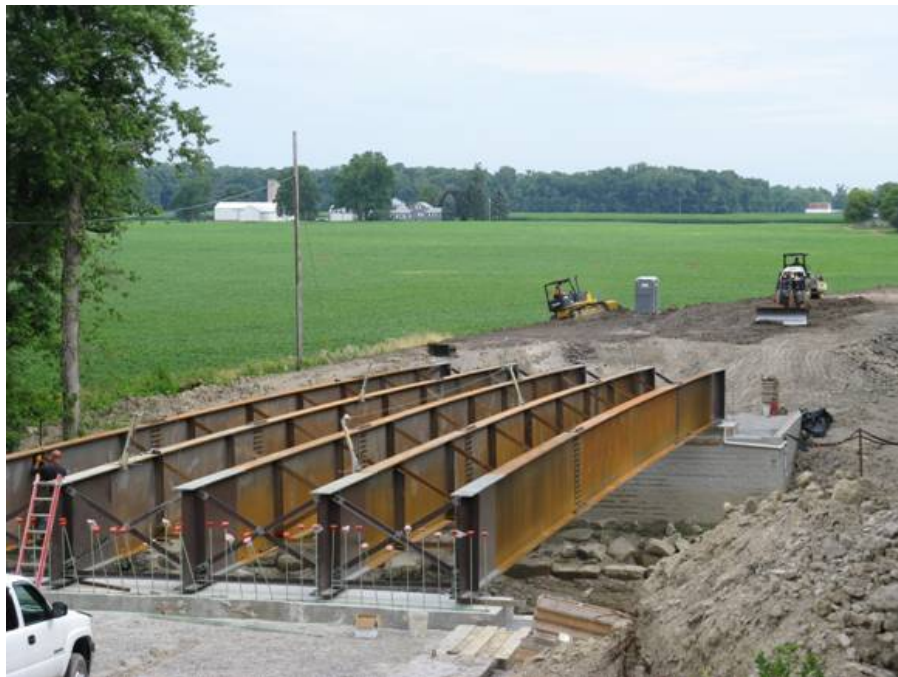
Figure 86. Photo. Steel girder on CIP footing.
