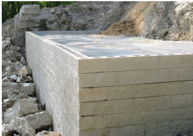
Figure 66. Photo. Right-angle wall corner.
