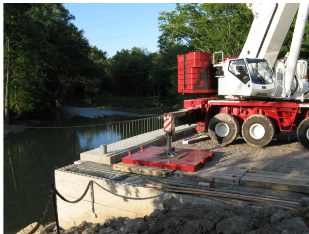
Figure 89. Photo. Outrigger pads near the wall face.
