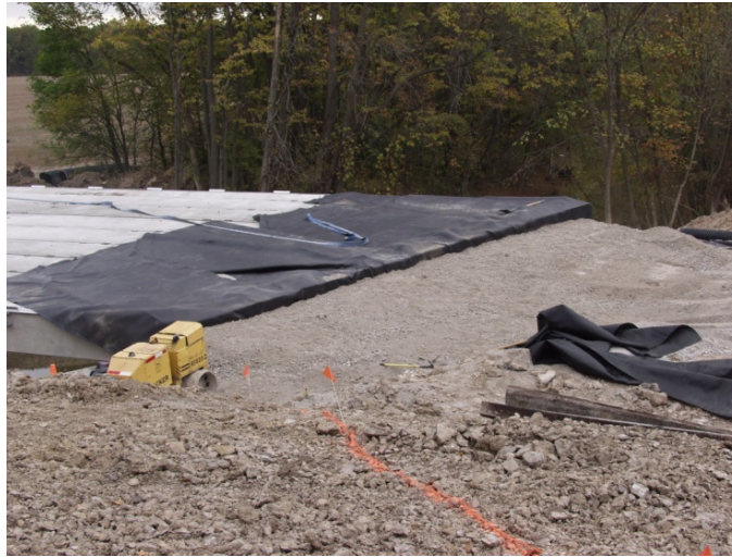
Figure 96. Photo. Second 6-inch-thick fill lift.
