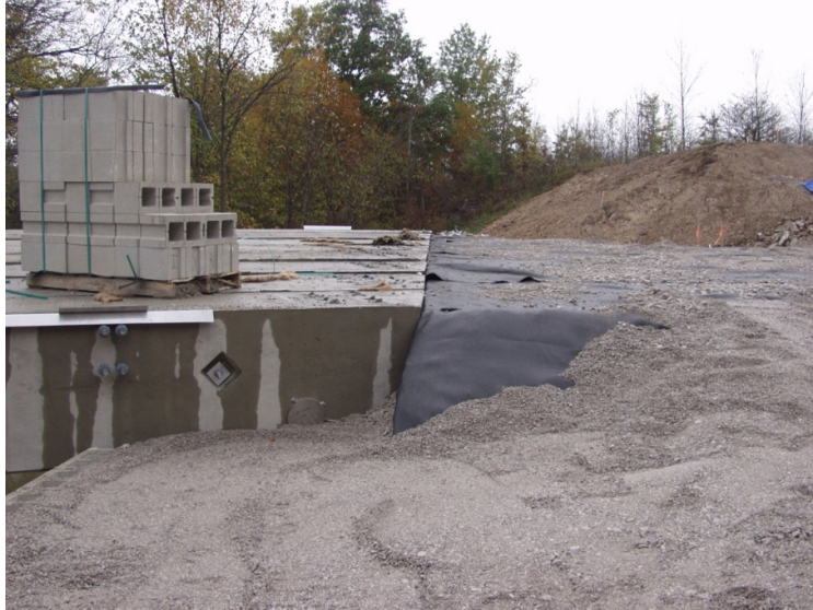
Figure 97. Photo. Completed approach fill.
