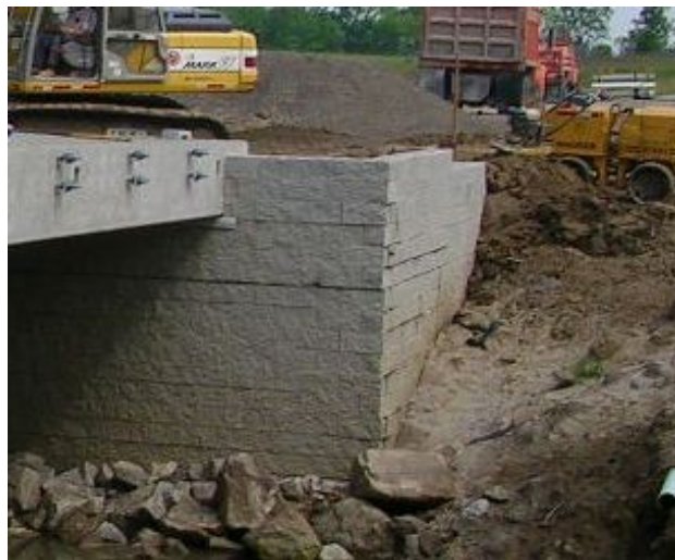
Figure 90. Photo. First view of parapet and wing wall construction.
