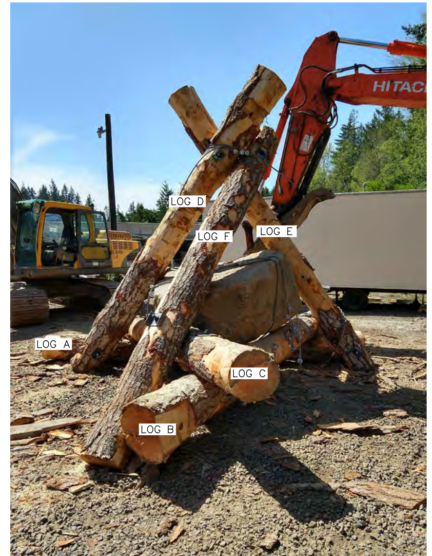
THE LOG JACK IN THE IMAGE ABOVE IS TYPICAL AND FOR ILLUSTRATION ONLY. DISCREPANCIES EXIST BETWEEN THE IMAGE AND THE LOG JACK DESIGN.
