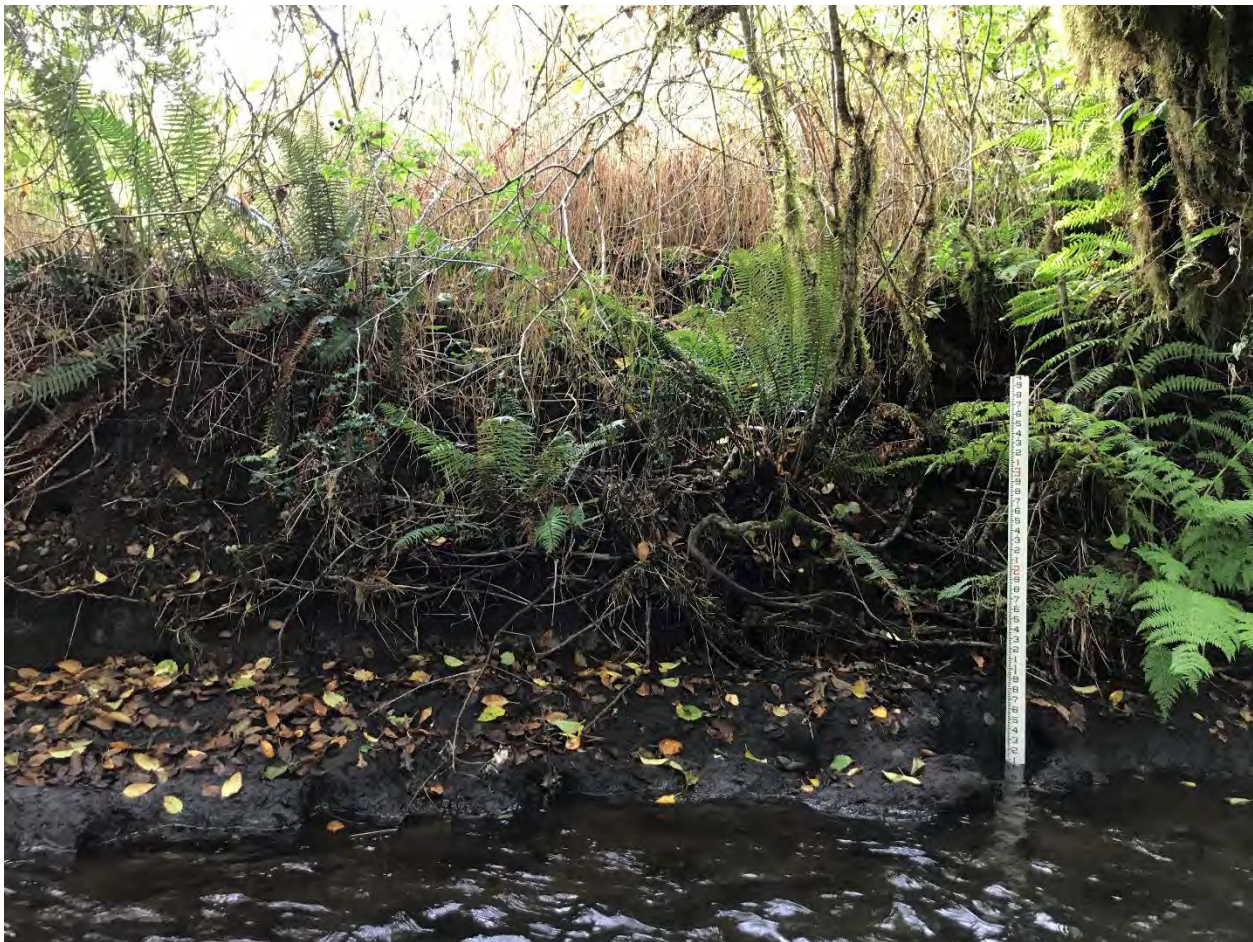
Figure 8 Down-cut banks downstream of Crumb Road expose mudstone and roots
