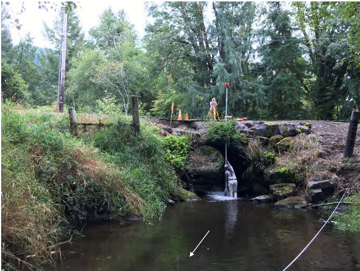
Figure 2 Existing conditions at the Crumb Road culvert outlet
