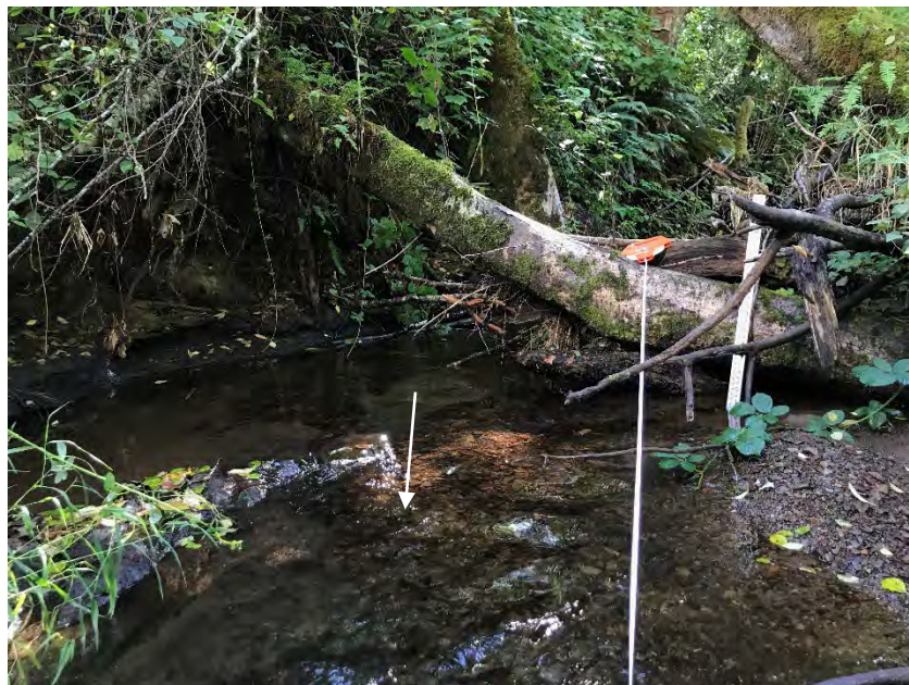
Figure 15: View of the channel bend upstream of the culvert inlet, with exposed mudstone bed, bank scour, and a debris jam forming on a large tree spanning much of the channel (Station 25+70, white arrow indicates flow direction)
