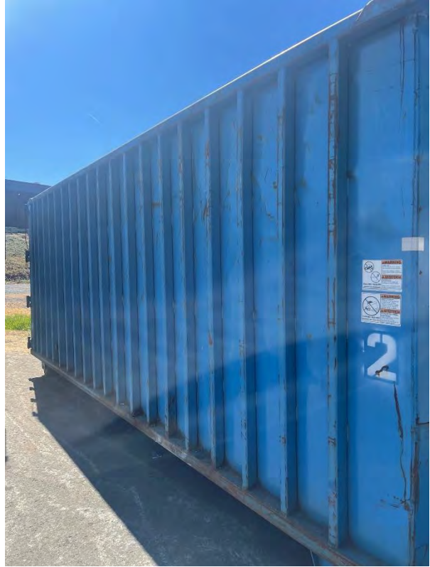
Figure 9: Vertical Reinforcing Members
