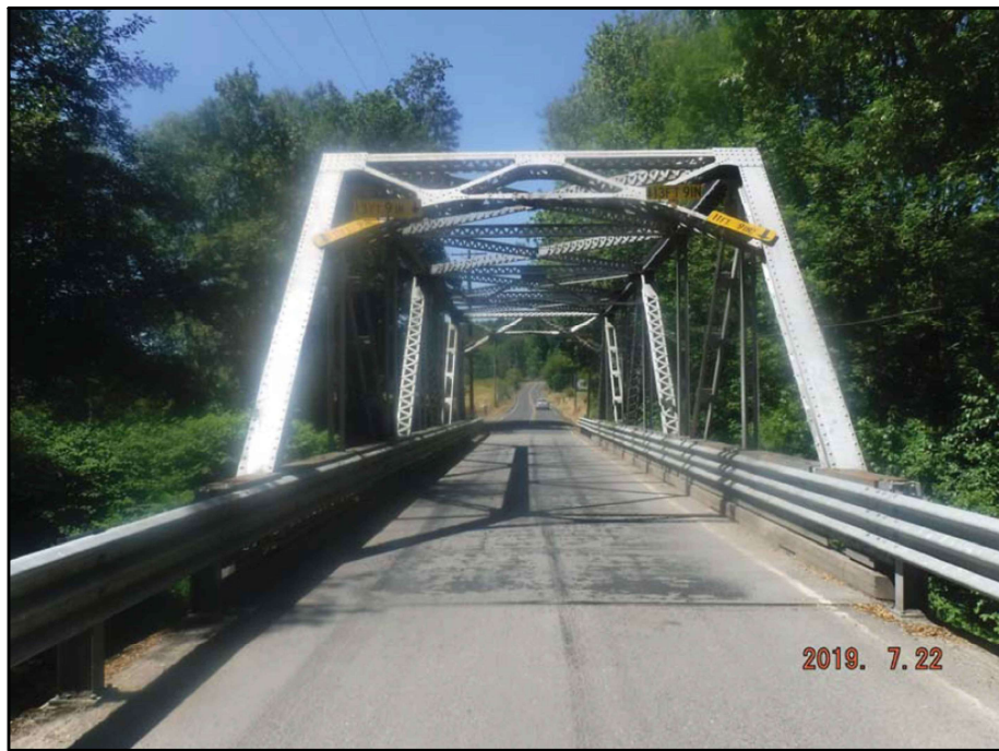
SI-25: EAST PORTAL LOOKING WEST
