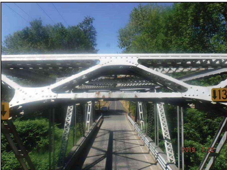
SI-36: U5 (EAST) PORTAL LOWER CHORD
