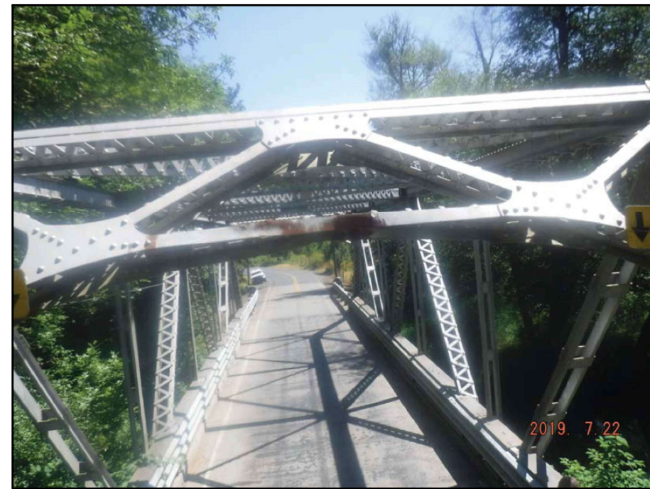
SI-26: U1 (WEST) PORTAL LOWER CHORD
