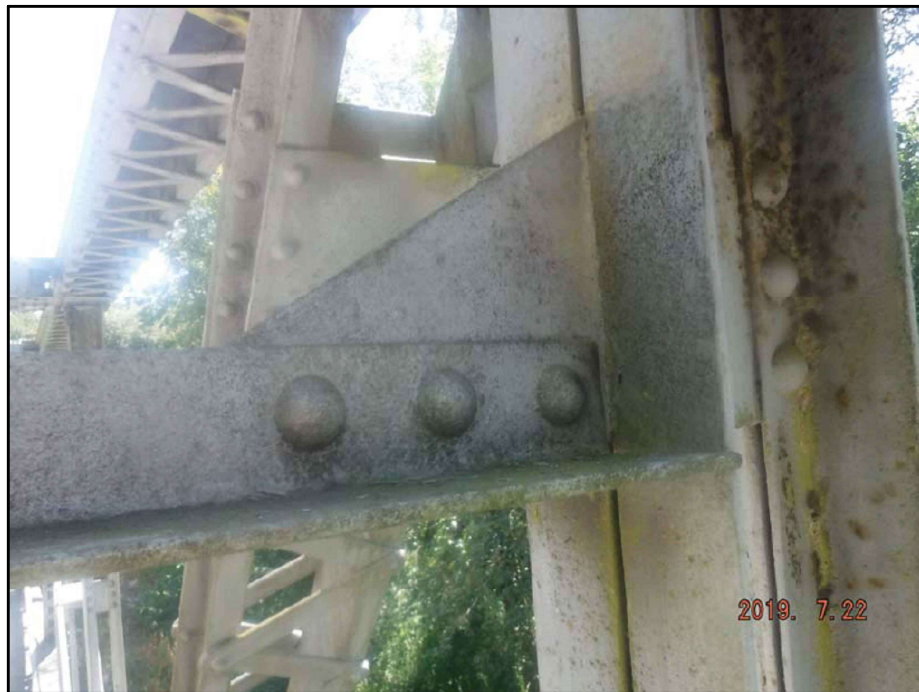
MS1-34: U3 SWAY LOWER CHORD KNIFE PLATE CONNECTION
